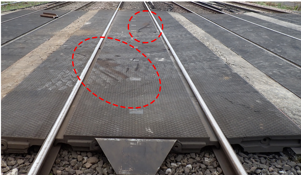
Figure 12: The witness marks (red dashed circles) caused by the section of rail impacting the rubber surface of the RRAP around the Up Fast line. Tyre marks on the RRAP surface, probably caused by the RRV on the 2 March, are also visible on the Up Slow and Up Fast lines.
