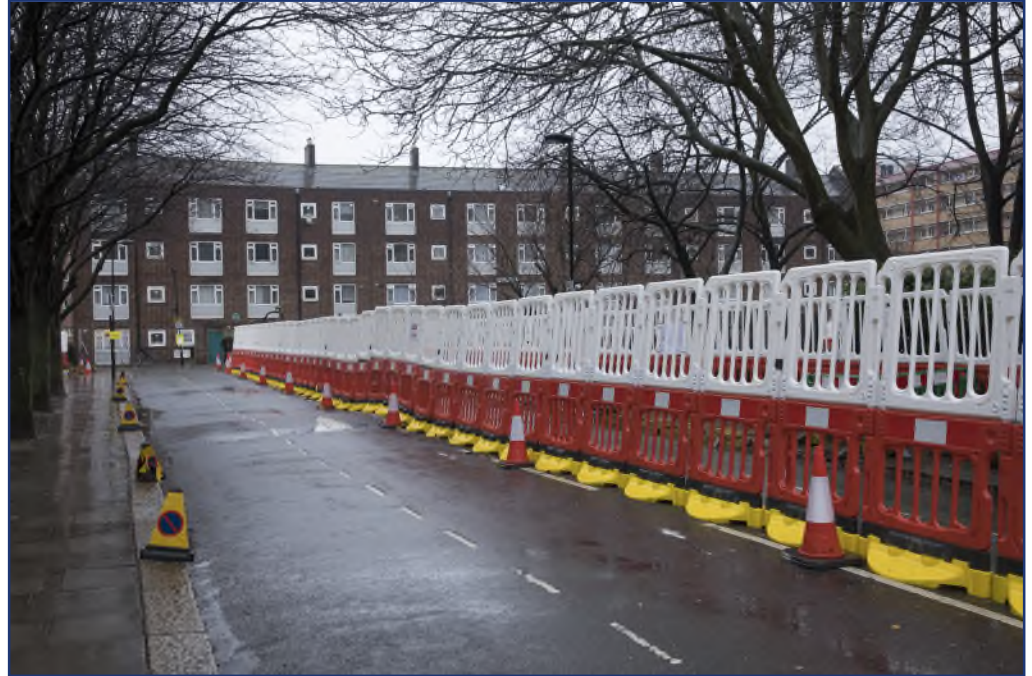
HS2 Phase One, works at Euston
