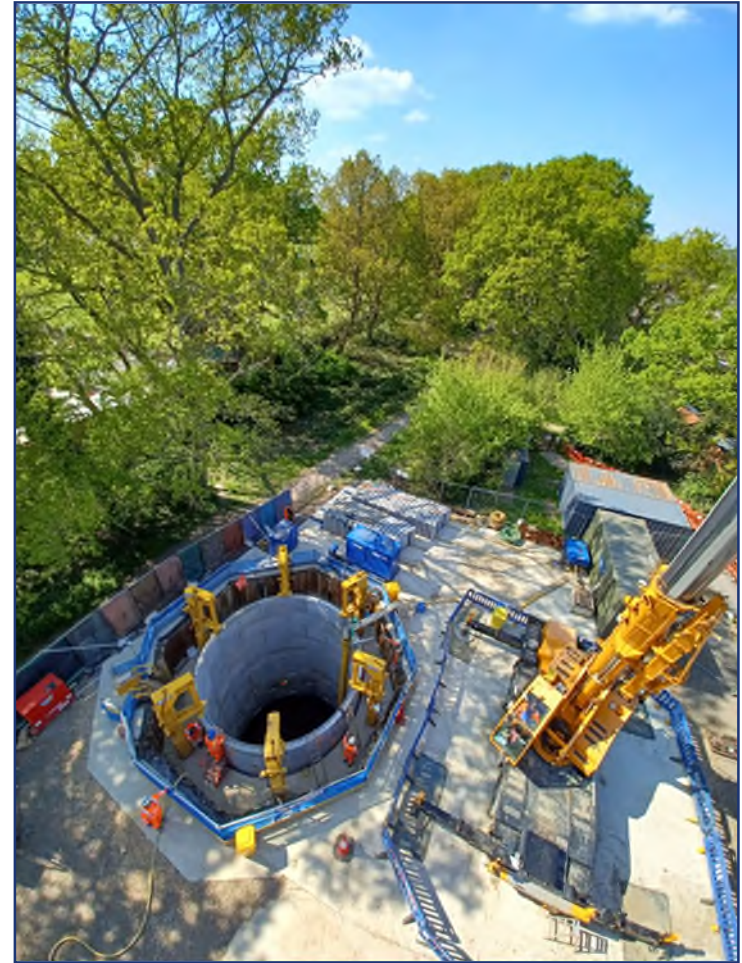
An access shaft for a TBM drive under construction at HS2 Phase 1 Thames Water Greenway site (West Ruislip), with precast rings jacked downwards, along with its dedicated crane and lifting platform.
