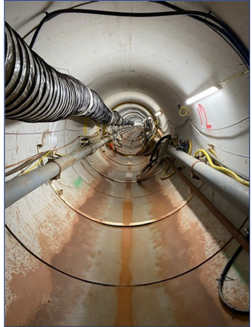
HS2 Phase One, 1800mm Sewer from the Erskine St Scheme in Birmingham under construction, with MTBM supply lines visible.
