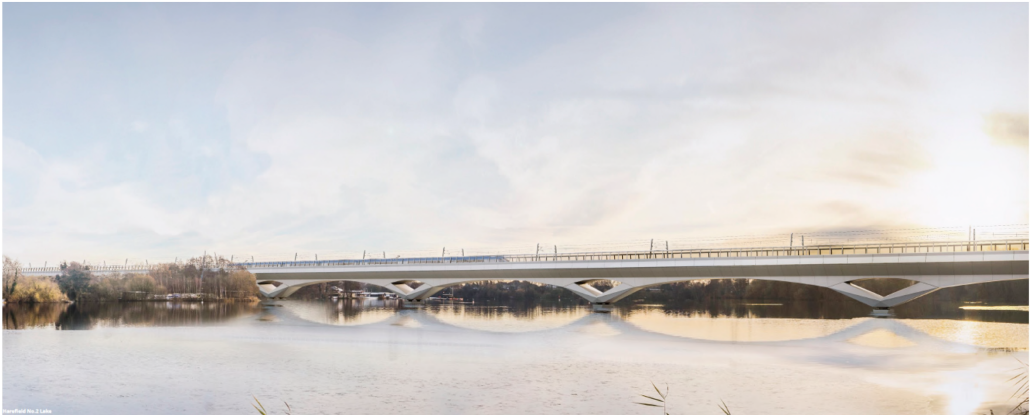
Colne Valley Viaduct
