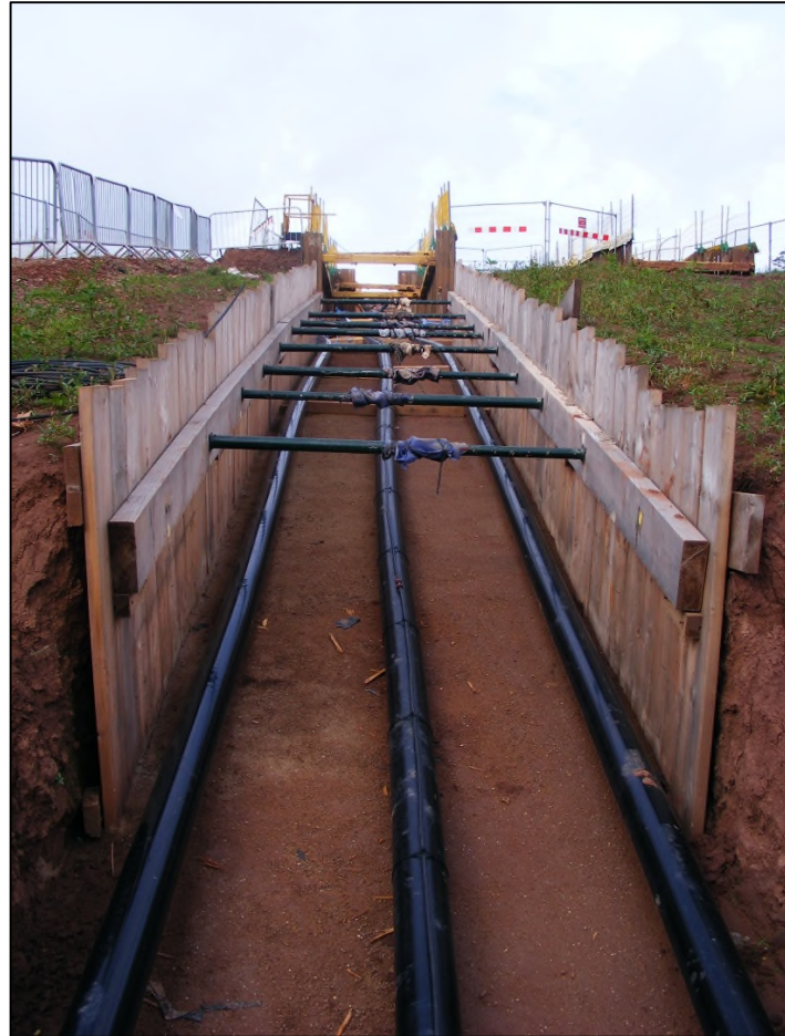
Installation of ducts ready for cabling
