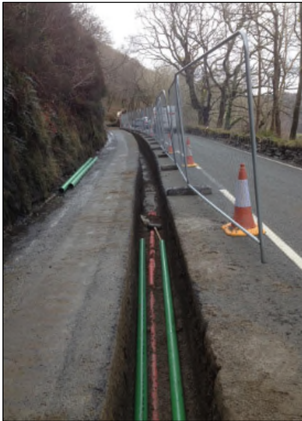
Works within single carriageways – traffic controlled
