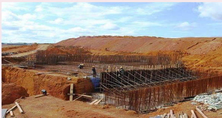
Nyumba Ya Akiba cement plant under construction in DRC. © EAI/PIDG
